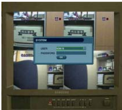
Picture of Power On after Finishing Installation
